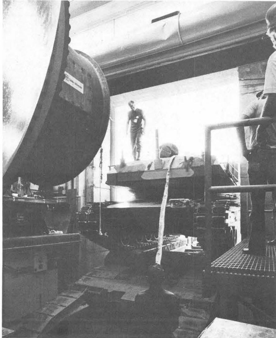
**HERMES II, MEET THE XM1** — This improbable liaison, between the Army's latest tank and Hermes II, Sandia's flash X-ray machine in Area V, took place because the Army wanted to perform radiation vulnerability tests upon the new machine. Bob Schuch and Jesse Harness of Beam Source Applications Division 4232 worked with the Army people to squeeze the 60-ton XM1 into the test area. The tank has a turbine engine, is based at White Sands.
